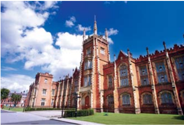
Fig 1. Queen's University Lanyon Building.
