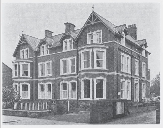
Figure 2. Alexandra Gardens Day Hospital
