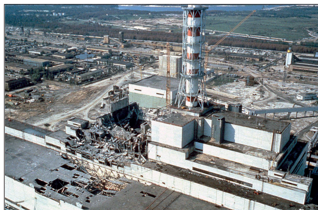
Fig 8. The destroyed reactor at the Chernobyl nuclear plant.
