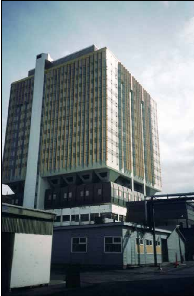
Fig 4. The completion of the West Podium Extension in 1984 (bottom right of picture just visible behind the black pipework).
